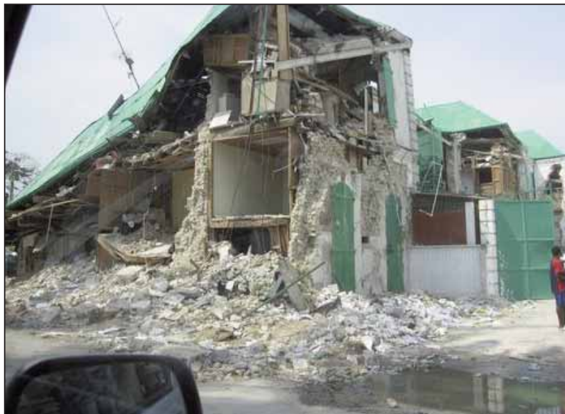
Scenes of the aftermath of the earthquake (above and below).
