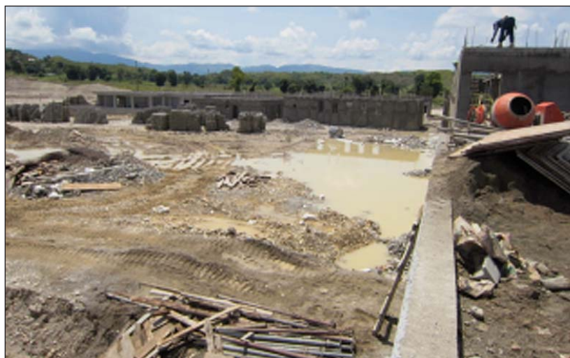
The future site of the operating rooms
